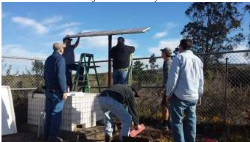
Removing the old Solar array
